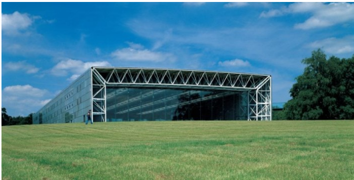
A LARGE HANGER AT NORWICH, UK (Foster + Partners, 1978). Width 34m, height 10m, length over 133m. The Nave of Notre Dame is 40 feet wide and about 107 feet in height. (Image via Nigel Young, dezeen.com)
