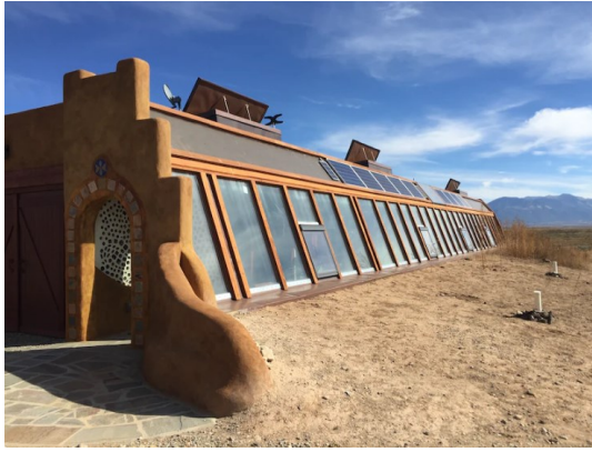
EARTHSHIP (JOHN WENZ, 2015) The walls do not carry any weight; the Trombe-window walls go right round the south of the House. (Image via Inverse.com)
